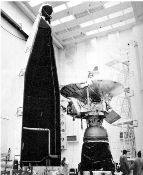
To ensure operational readiness of the spacecraft and its science instruments for launch, it was tested through a simulated countdown in Building AO (Figure 5-2). The RTGs were installed and the spacecraft loaded with propellant. Finally, it was mated to the third stage of the launch vehicle and encapsulated within a protective nose shroud for its journey through Earth's atmosphere. The entire assembly was then transferred to the launch pad and mated to the Atlas-Centaur.
